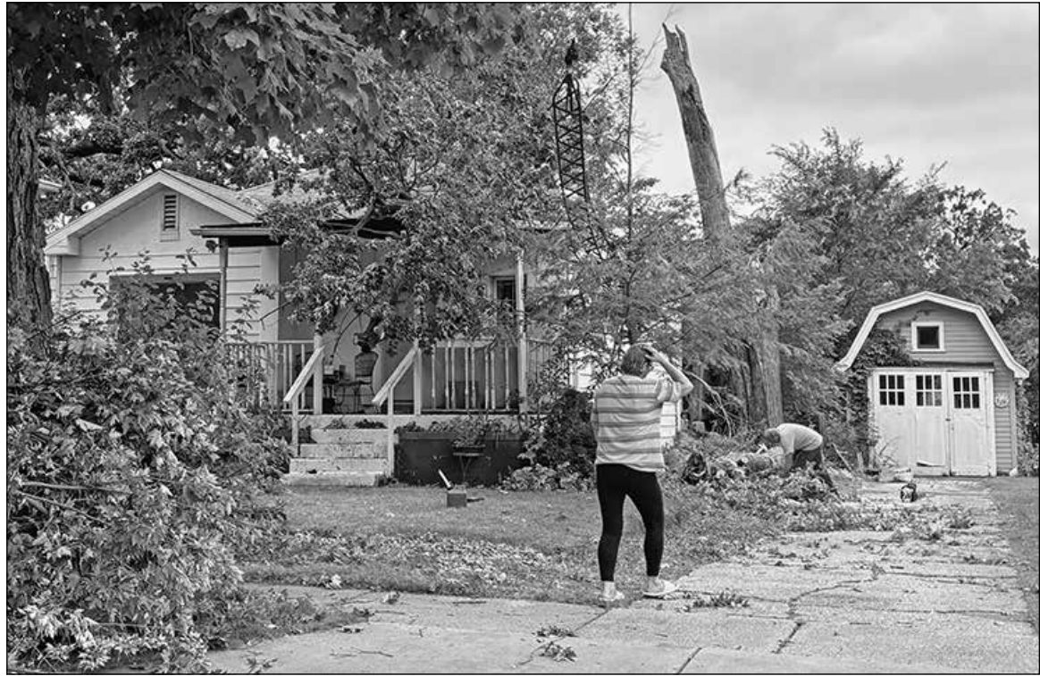
While there was no tornado in Delavan, damage from the storm was evident. This house near the historic downtown area of the city had both a tree and an old antenna tower fall on it.
